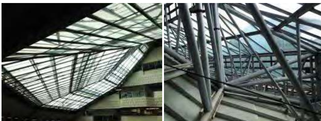
Figure 7: Glazed, double-skin roof of the library
