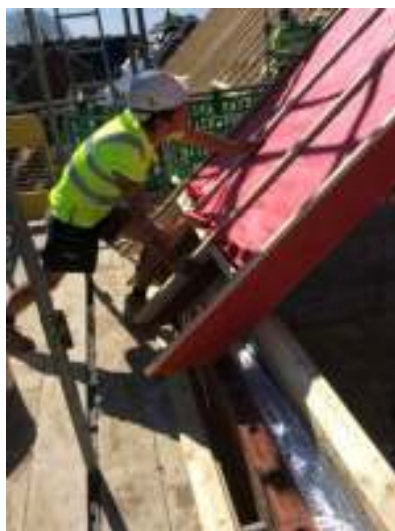
Figure 8: Tradesman installing one of the prefabricated roof panels.
