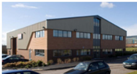
Fig. 1. Picture of the case study building.
