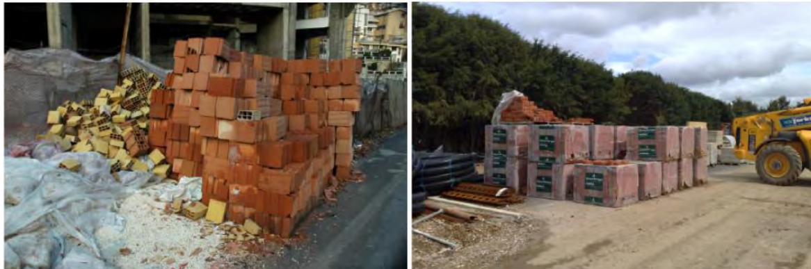
Figure 4: Construction material storage and waste in Iran (left) and the UK (right).
