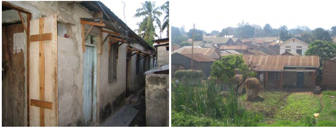
Figure 1: low-income housing with iron sheet roofing.
