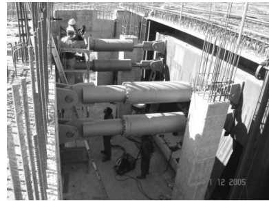
Fig. 2.3 Fluid Viscous Dampers for De Las Piedras-High Speed Railway Bridge, Spain [Courtesy of Maurer Sönbe, Germany]
