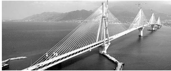
Fig. 1.4 Rion-Antirion Bridge, Greece [from www.aecom.com ]
