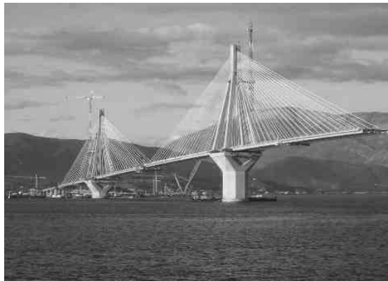
Fig. 2.23 General View of the Rion-Antirion Bridge [Infanti et al , 2004]
