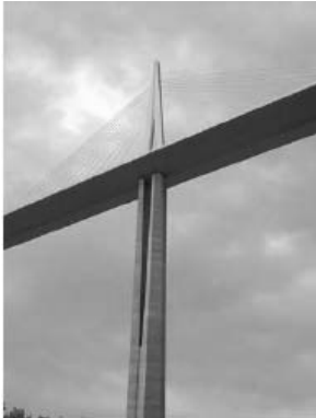
Fig. 1.16 Millau Bridge, France
