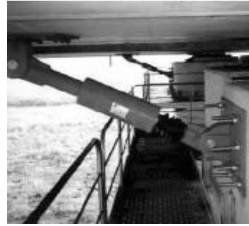
Fig. 2.9 850 kN Capacity Damper for the Chun-Su Bridge, South Korea [Courtesy of FIP Industriale s.P.a. , Italy]
