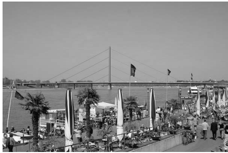
Fig. 1.9 Oberkassel Bridge, Düsseldorf, Germany
