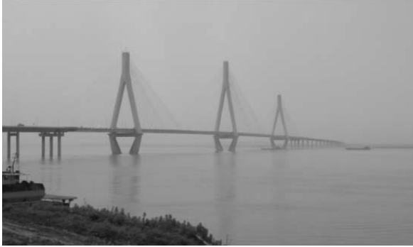
Fig. 1.19 Dongting Lake Bridge, China
