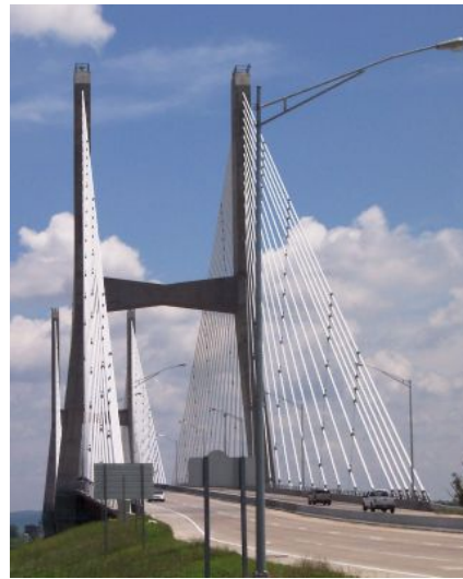
Fig. 6-31 Vista general del puente Memorial Bill Emerson
