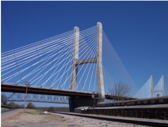
Fig. 6-30 Vista general del puente Memorial Bill Emerson
