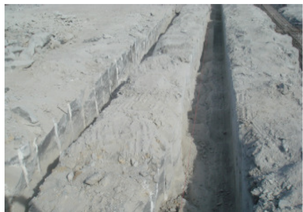
Fig.39,40 Unnecessary pollutant excavation in hard rock due to the application of criteria corresponding to soil.
