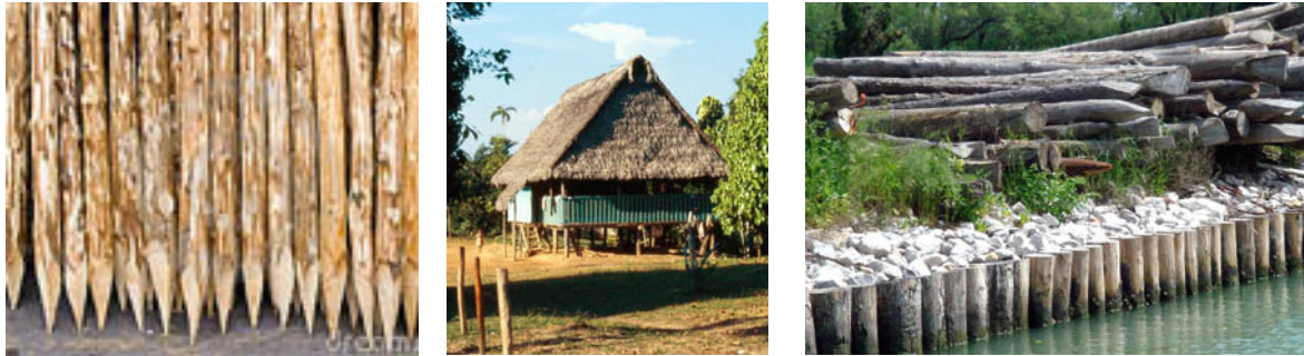
Fig.1,2,3: Timber piling is the oldest foundation system, extensively used in many applications. It has recently emerged as a low-energy, cost-effective sustainable solution (fig.1,2,3 and: http://www.geoforum.com/info/pileinfo/view.asp?ID=56 )
