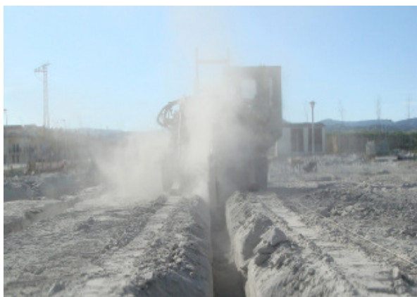
Fig.39,40 Unnecessary pollutant excavation in hard rock due to the application of criteria corresponding to soil.
