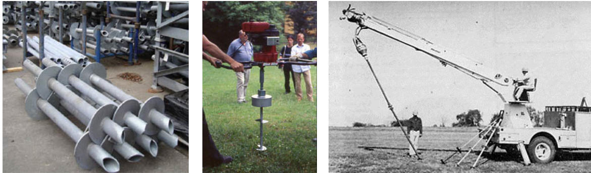
Fig.26,27,28: Screw piles are manufactured using varying sizes of tubular hollow sections. They are installed using earthmoving equipment fitted with rotary hydraulic attachments.
