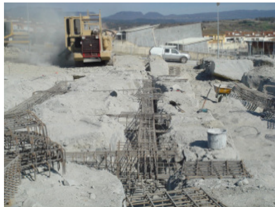
Fig.41,42 Useless excavation and reinforced tie beams intended to brace the footings in hard rock.
