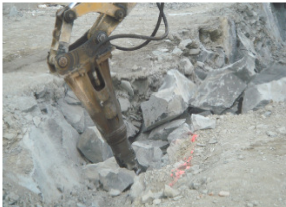
Fig.41,42 Useless excavation and reinforced tie beams intended to brace the footings in hard rock.
