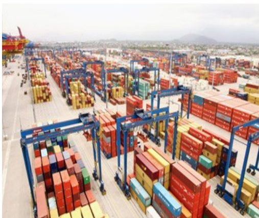
RTG Cranes (Yard)
