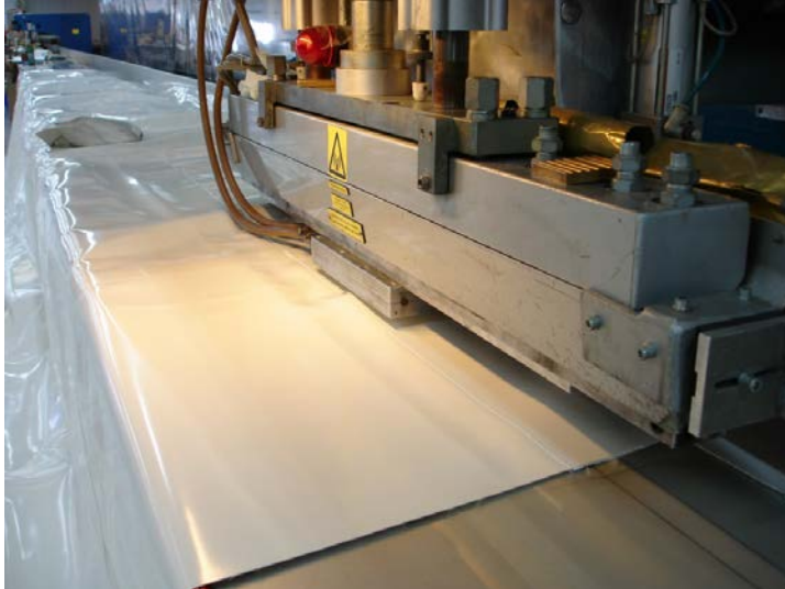
Figure 9-2 Typical welding situation [© CENO Membrane Technology GmbH]
