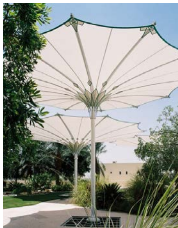
Figure 6-1 Membrane partly reinforced with a second layer at the low point and membrane corners [© Ceno Membrane Technology GmbH]
