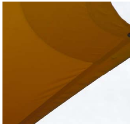
Figure 7-4 Slight wrinkles in a corner detail [© R. Koenen]
