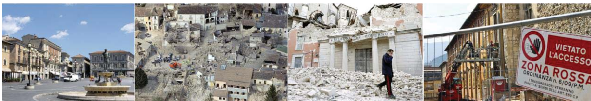
Figure 1: Historical city centre of L'Aquila before and after the 2009 earthquake
