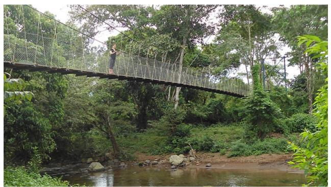
This safe and resilient B2P bridge sits high above a non-flooded riverbed, but note that the high water mark is approximately a metre and a half back from the water's edge and roughly a metre higher (© 2021, Kevin Donovan)
