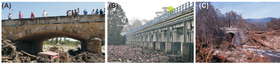
Figure 1. Partially clogged bridges with large wood and drift material crossing the Rivers (A) Seco (Teruel), after the August 2013 flood (source: ABC online newspaper); (B) Nalón (Asturias), after the 2012 flood (source: La Nueva España online newspaper); (C) Cabrera (Ávila) after the 1997 flood (this event is described in the text).
