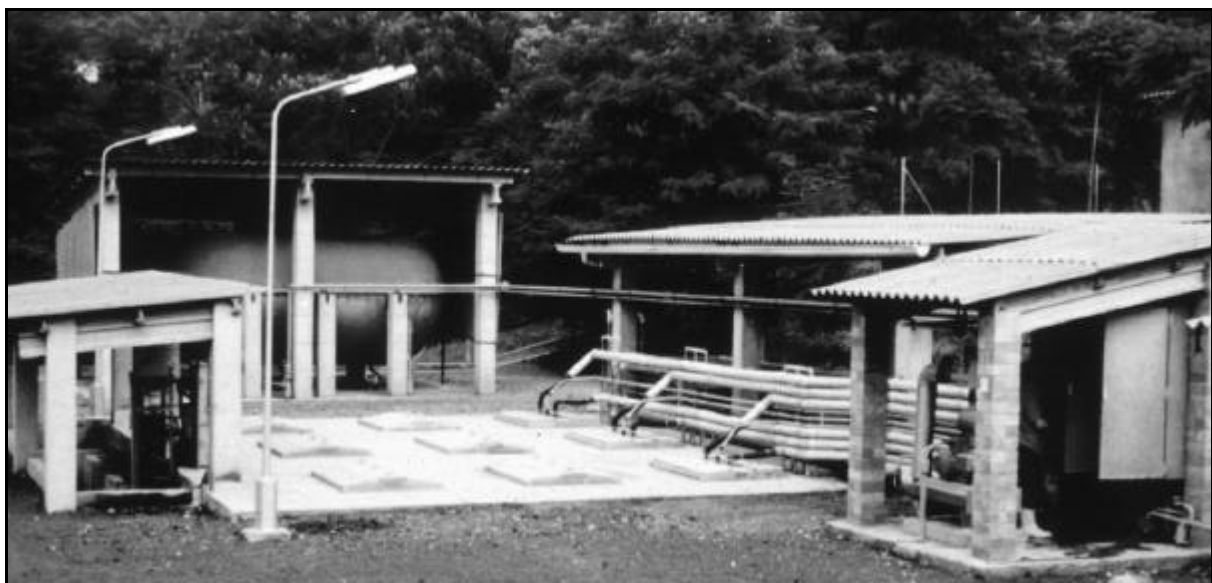
Fig. 2.- A view of Mas El Cros biogas plant
