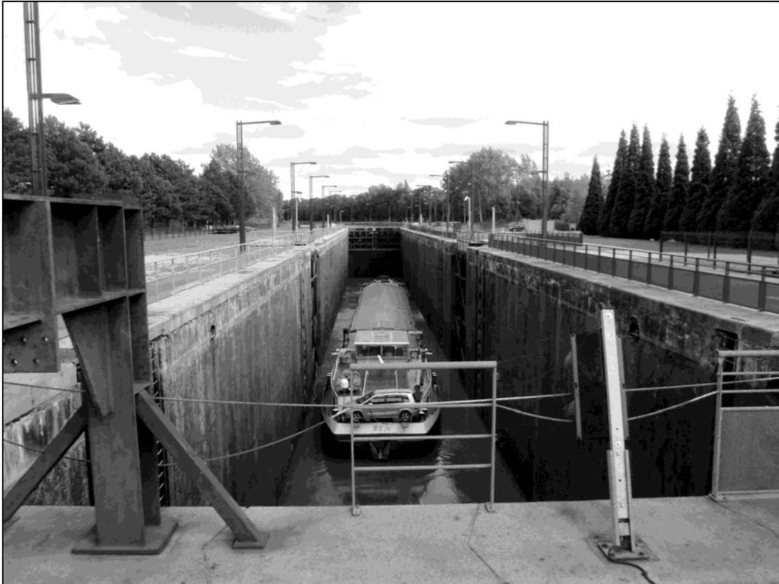
Figure 3: A ship inside the downstream lock (Fontinettes) during the filling process.
