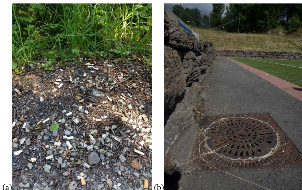
Figure 4. High amounts of tire crumb are visible on the southern footpath between the artificial turf field and the stream Drengsrudbekken (a), drains next to the turf field are lined with geotextile (b).
