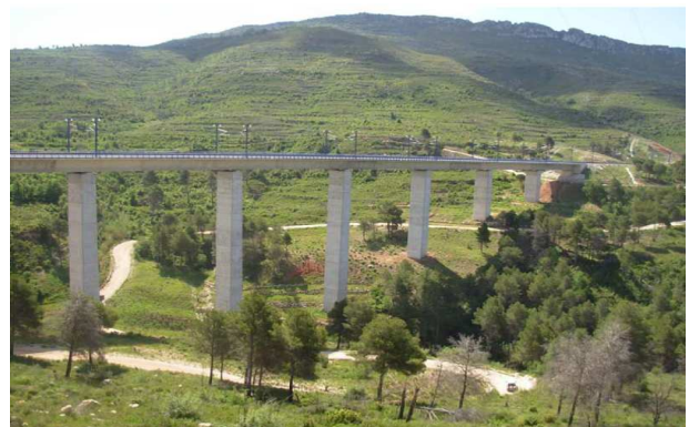
Figure 1. General view of Pont de Candí Bridge in Dec. 2007
