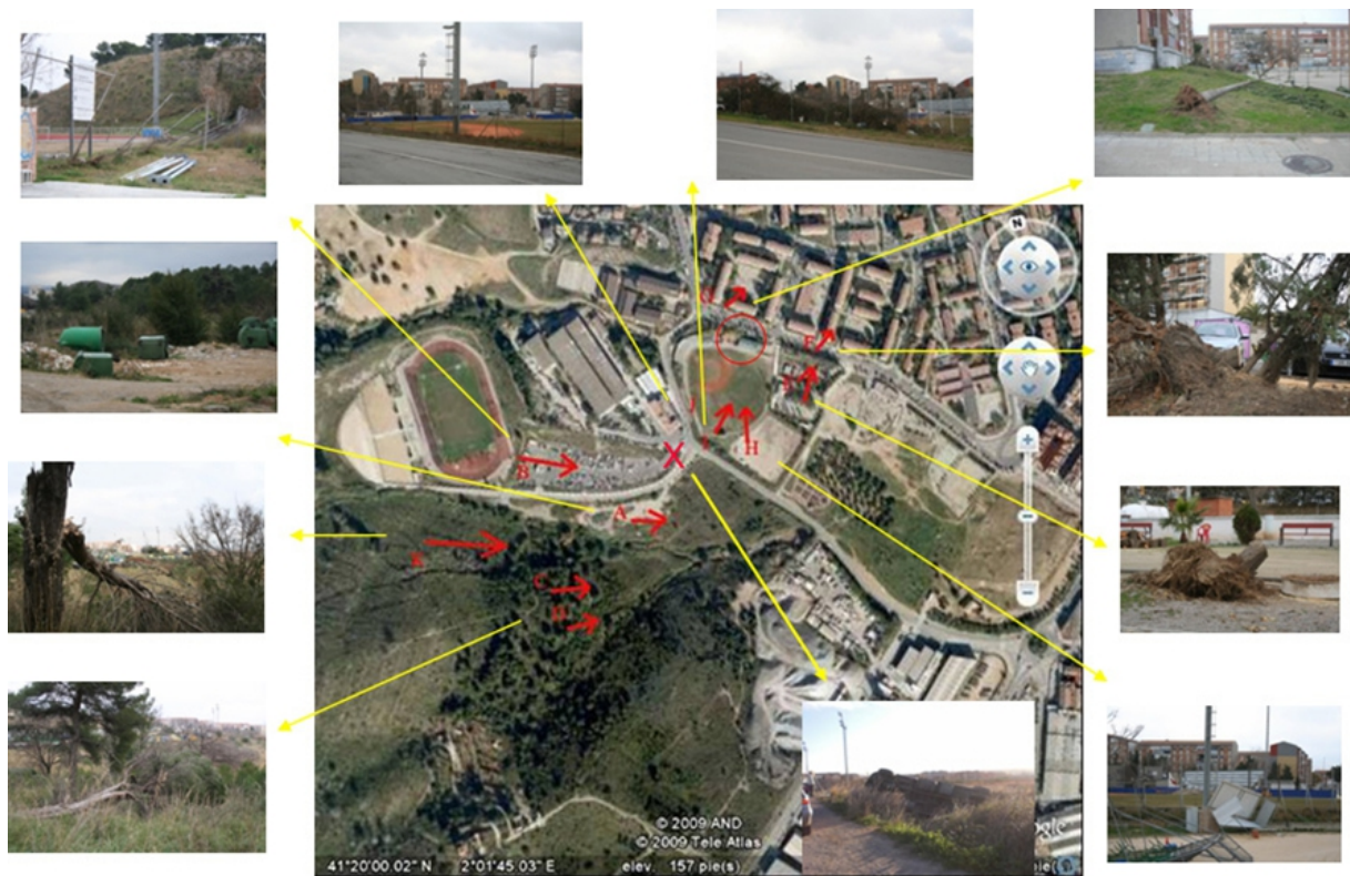
Figure 7. In situ analysis of the damage around the facilities of the Sant Boi baseball camp. The red circle indicates the location of the collapsed facility. The red arrows indicate the direction (not the intensity) towards which the different strewn elements were found. The small pictures indicate those elements.
