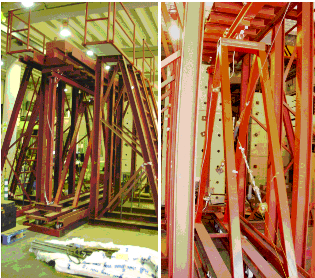
Figure 2. Left: The portico used to study the damping effect of SMA damper, the figure shows the lateral protections that avoid the out-of-plane oscillations. Right: The SMA dampers were situated in the portico diagonals and completed by steel wires. The reaction wall for the hydraulic piston is situated in the portico rear.
