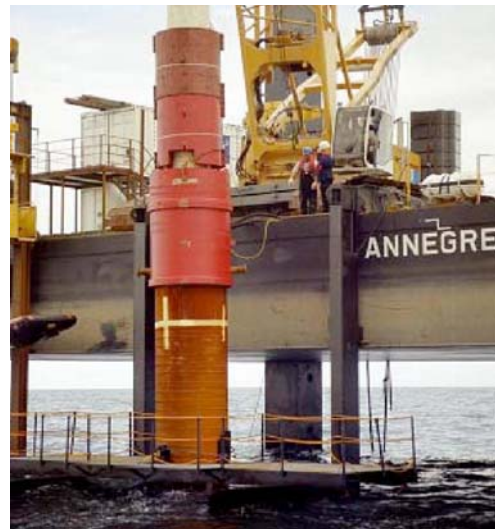
Fig. 1 Pile driving process. [2]
