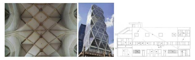
5.-A vault as the result of an intersection of volumes may be understood as simple, but in this case the addition of some ribs shows the diagonal connections between a column of an arch and the keystone of another. Those lines make explicit the exactitude and restrictions present in this particular configuration, and make it more structured and complex. *Graz cathedral*.
