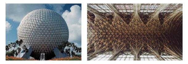
29.-The polyhedra that served as a base to this geodesic dome is so masked that possibly we are not aware of the hidden icosahedron. The pattern inside the faces of this polyhedron is a simple configuration of triangles which are integrated with the little triangles of the next triangular face; therefore the dividing edges between faces are lost. *AT&T Pavilion* by Buckminster Fuller.
