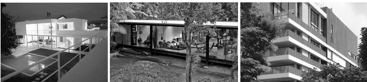
Figure 7: Veranda design strategies: interconnection, verandas that can be opened out or closed and verandas in vertical apartment blocks.
