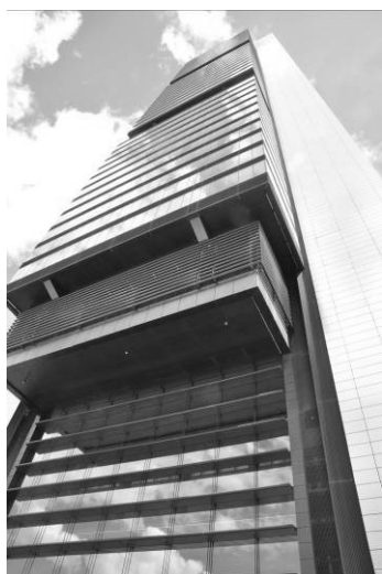
Fig. 12. Caja Madrid Tower. (Madrid)
