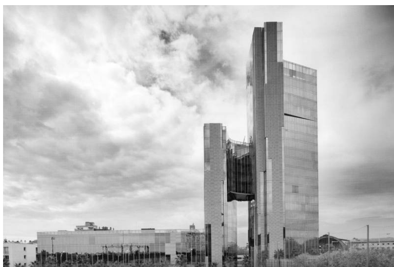
Fig. 13. Headquarters of Gas Natural (Barcelona). Ed. Pencil
