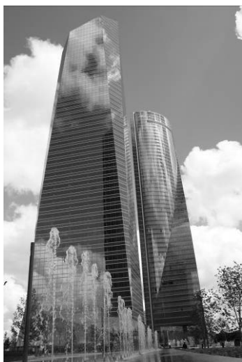
Fig. 01. Glass Tower. (Madrid)
