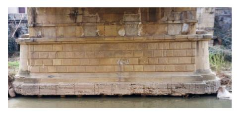
Figure 5 : Picture of the pier where piles are partly visible between the pile-cap and the water level.
