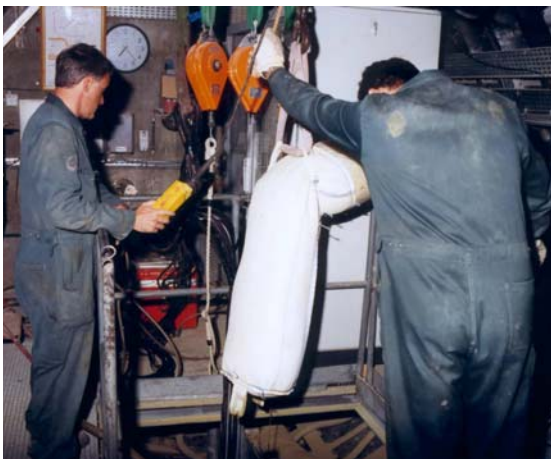
Figure 4-7: Installation of the seal: dumping the FoCa mixture in the shaft (left) and a top view of the shaft during installation (right).
