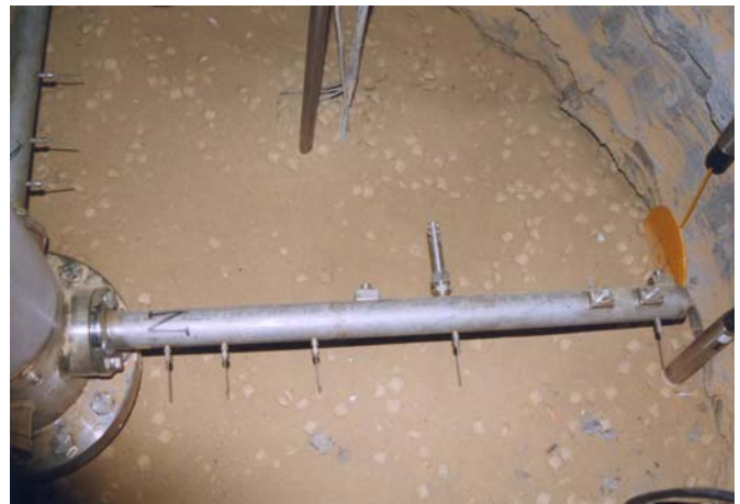
Figure 4-7: Installation of the seal: dumping the FoCa mixture in the shaft (left) and a top view of the shaft during installation (right).
