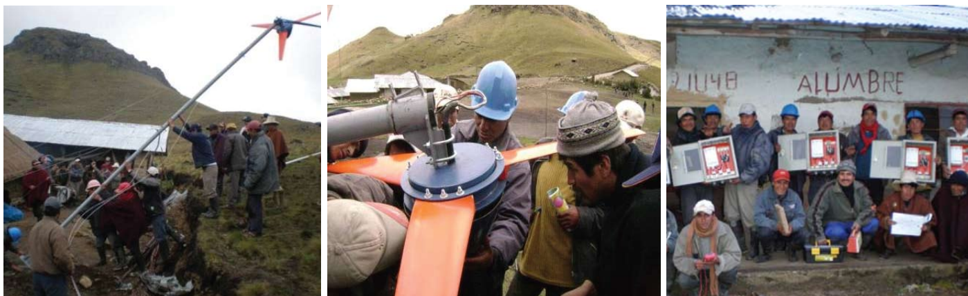
Figure 3. Installation process of the turbines and the battery controllers.
