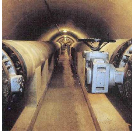
Figure 2: Drinking Water Network Pipes. Taken from [11]
