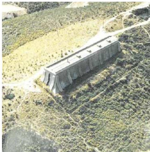
Figure 3: Barcelona Drinking Water Network Storage Device. Taken from [11]
