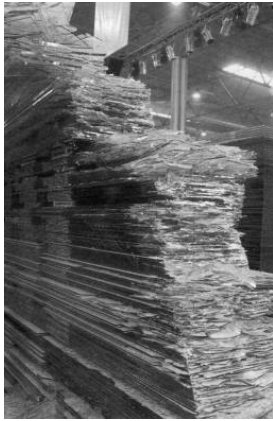
Waste sheet glass, piled up to form a load bearing wall.
