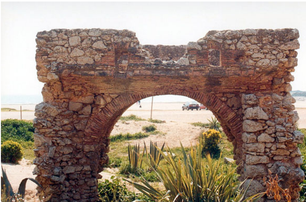
Figure 10. Note the holes in the wall of the pond room prepared for two waterwheels. From the information available, only one wheel and one set of millstone were installed.
