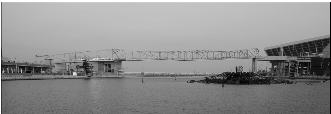
Fig. 13. Longitudinal view of the completed footbridge. On the right the Marina Seca slab. On the left the Capitanía building
