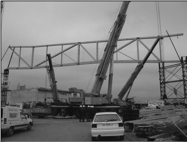
Fig. 7. Lifting of the first truss segment
