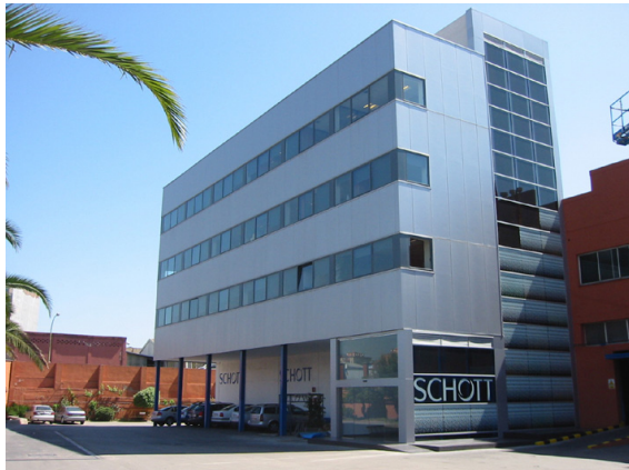
Figure 9: Outside view of finished façade.
