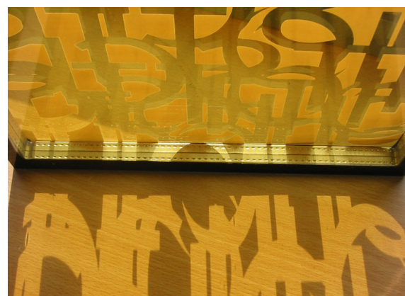
Figure 5: Double-glazed IMERA element with screen-printing as sun protection and design feature.
