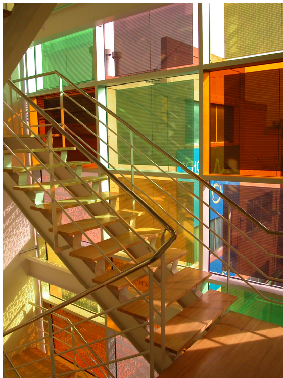
Figure 10: Inside view of finished façade.
