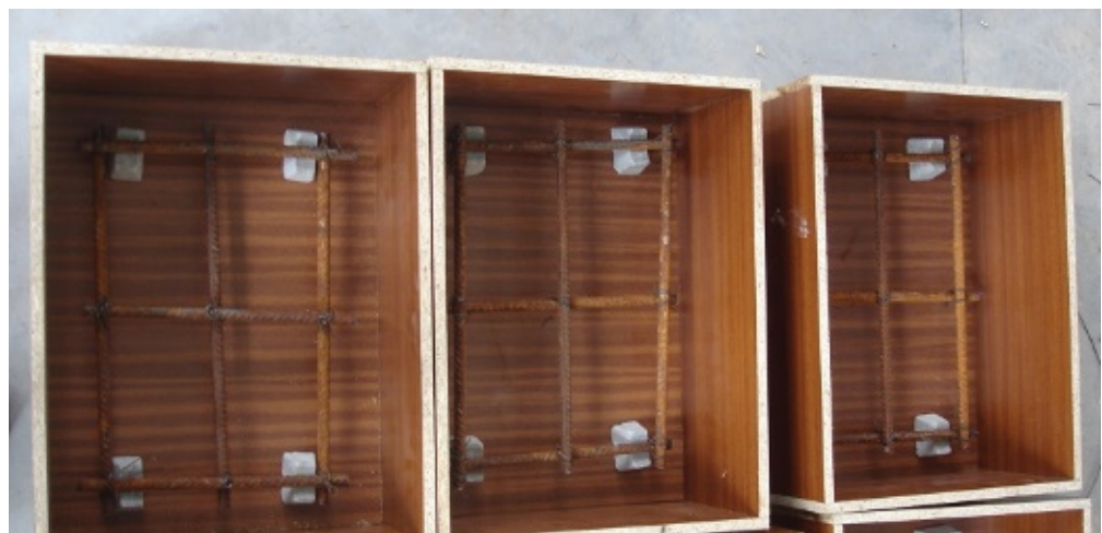
Figure 1: Preparation of samples for concreting.
