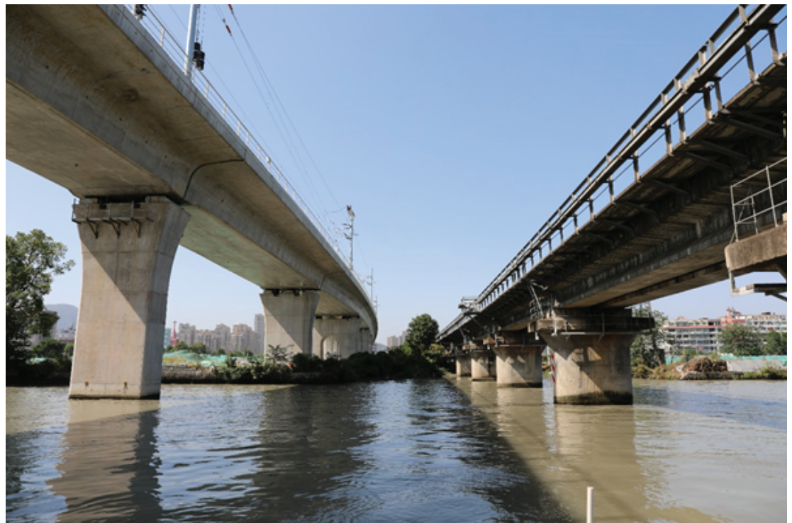
Figure 3: Train and light rail crossing the Wenruitang. (Photo:Wang Yue).
