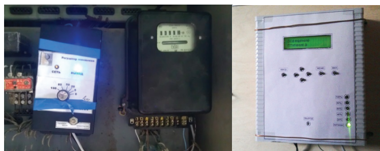
Figure 8: Testing a lighting system connected to an electric meter
