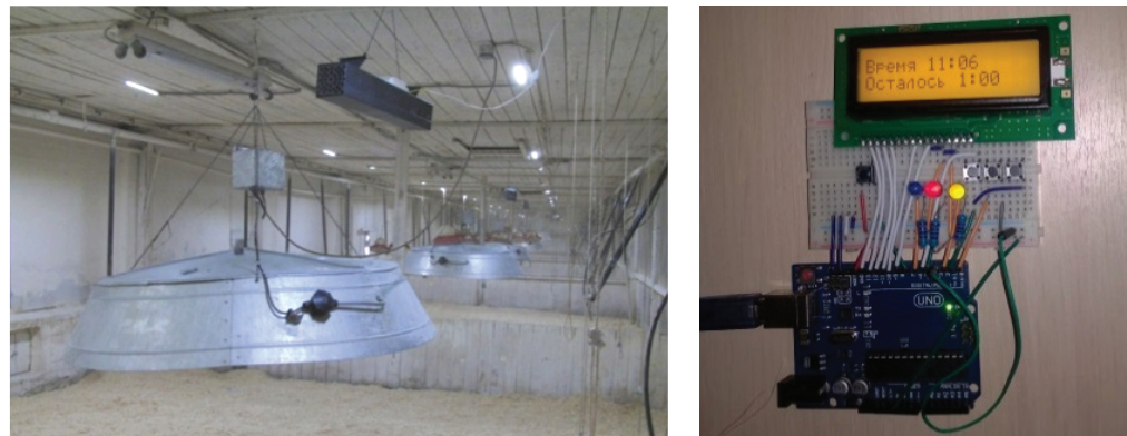
Figure 2: Lighting system testing
