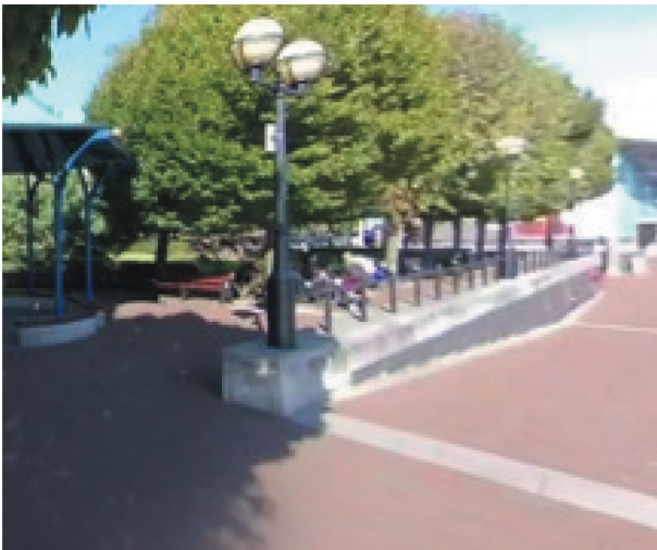
Figure 16. Retaining wall following natural terrain, Manchester. Possibility to shorten the route by stepping down.
