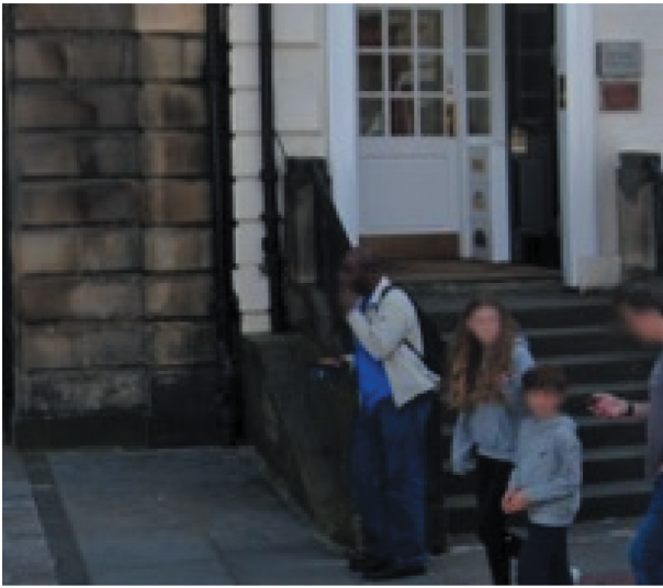
Figure 15. Entrance porch, Edinburgh. Possibility to step down on the side.
