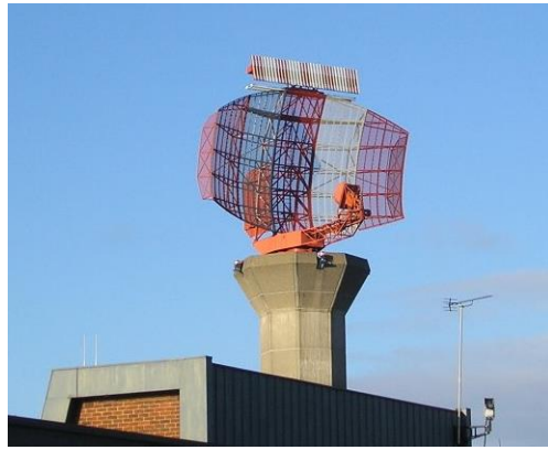
(b) Surveillance Radar (London Heathrow Airport)
