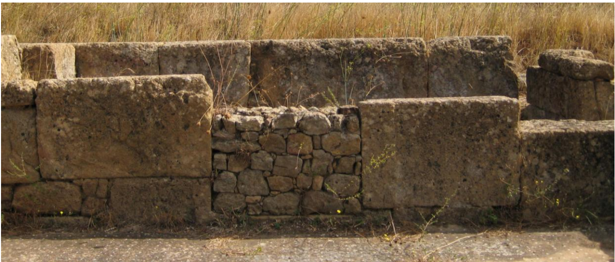
Fig. 4.19 Detail of the blocked up doorway between rooms 2 and 3 of Phase 2 of the House of the Official, Morgantina (author, September 2014).
