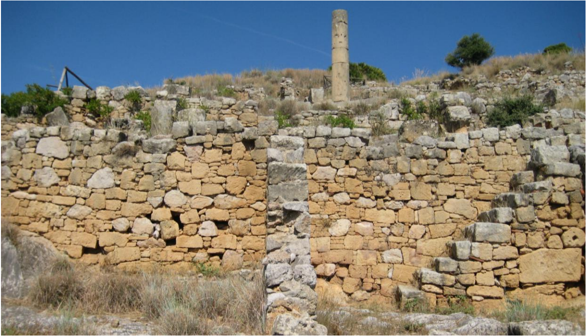
Fig. 4.20 Detail of retaining wall construction at Solunto (author, August 2015).
