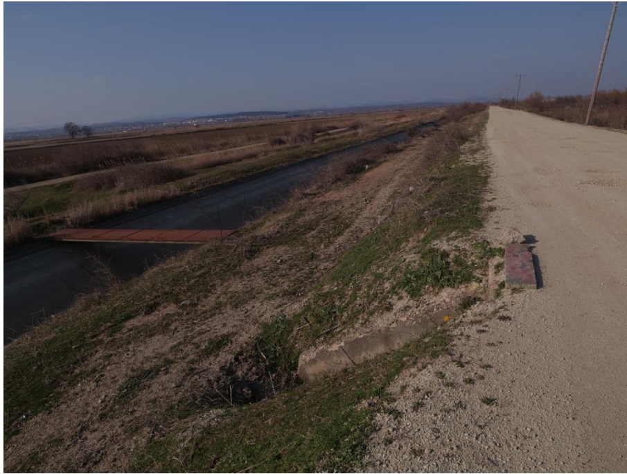
Irrigation works at the Delta near Feres.
