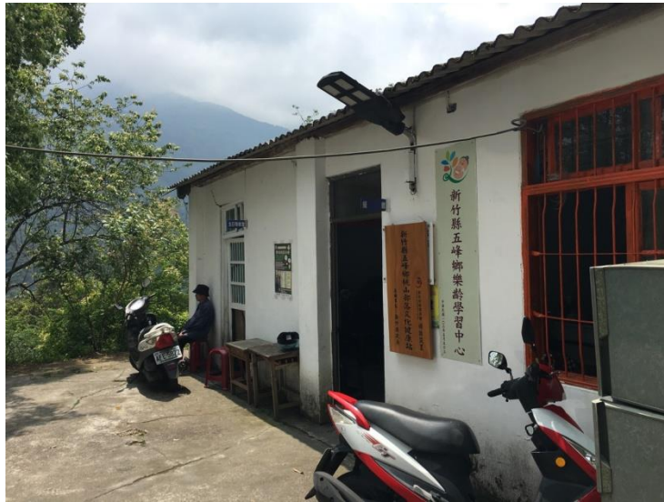
Figure 3. 4 Tribal Culture and Health Station in Taoshan Village, Wufeng.
