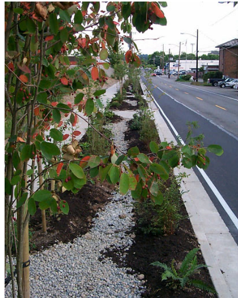
圖 2. 西北第 30 街的滲透性輸水溝渠 Figure 2. Permeable conveyance trench in 30 th Ave., N.E.
