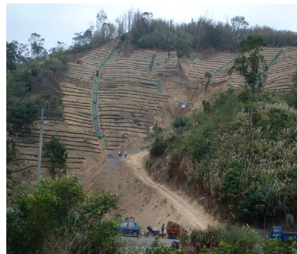
圖 8b. 崩場地處理現址-施工中(三灣鄉) Figure 8b. During construction.
