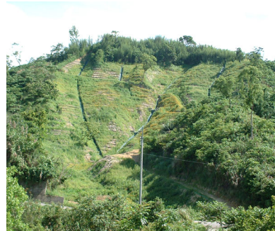
圖 8c. 崩場地處理現址-施工後(三灣鄉) Figure 8c. After construction.
