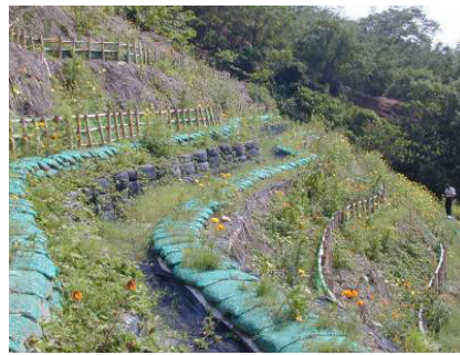
圖 7d. 坡面背填土袋橫向排水與植生 (5) Figure 7d. Backfill-bags for lateral drainage and vegetation on slope surface (5).
