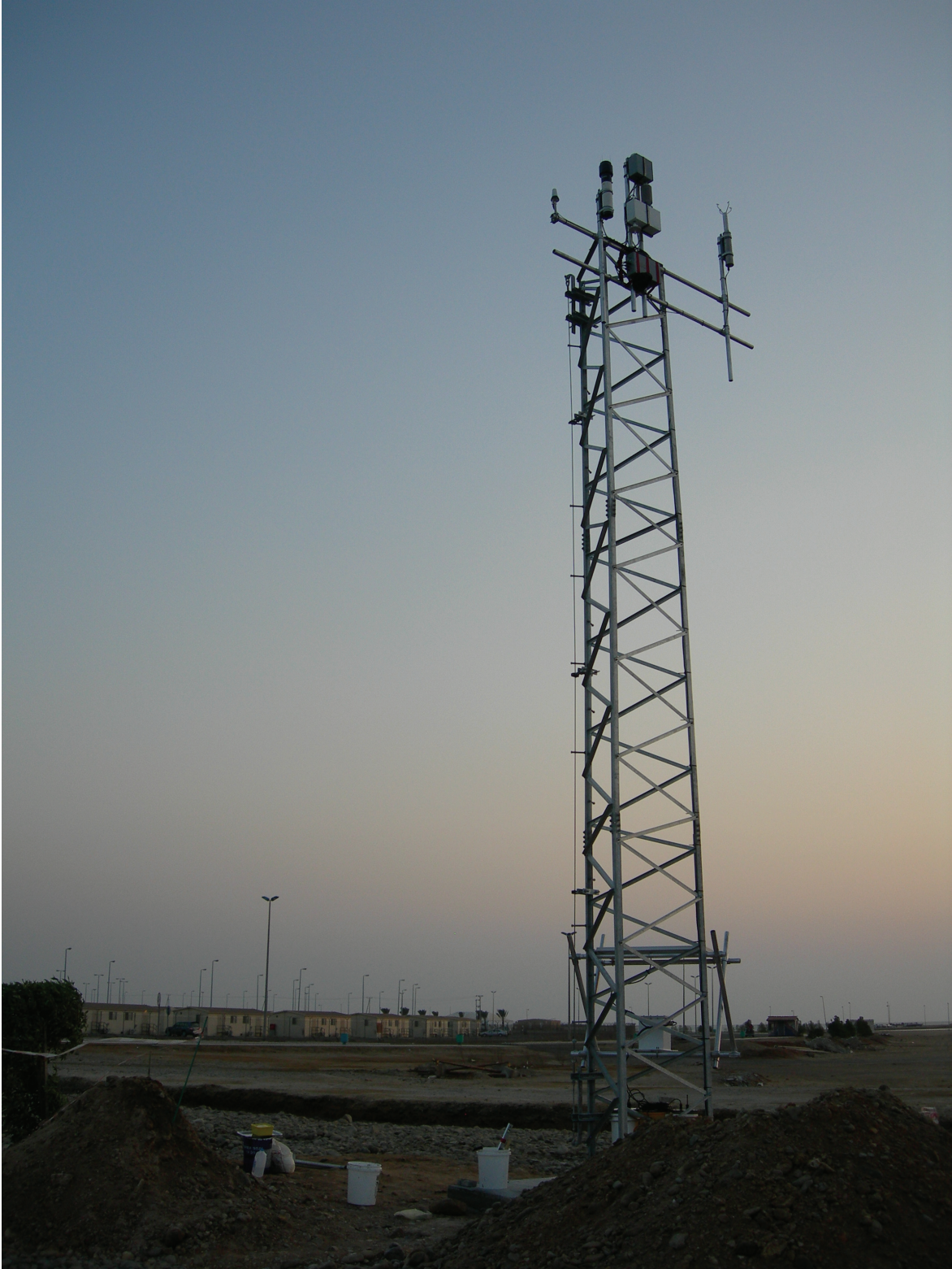
Figure VI-5: The meteorological tower after installation of instruments, telemetry system, and power system.
