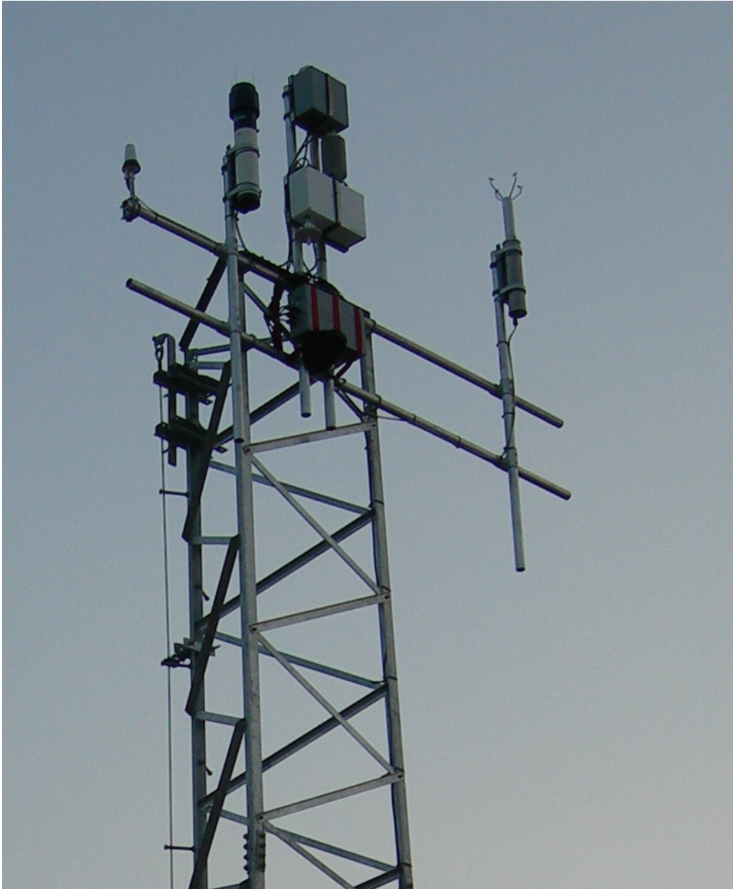
Figure VI-6: Close-up photo of meteorological system after installation.
