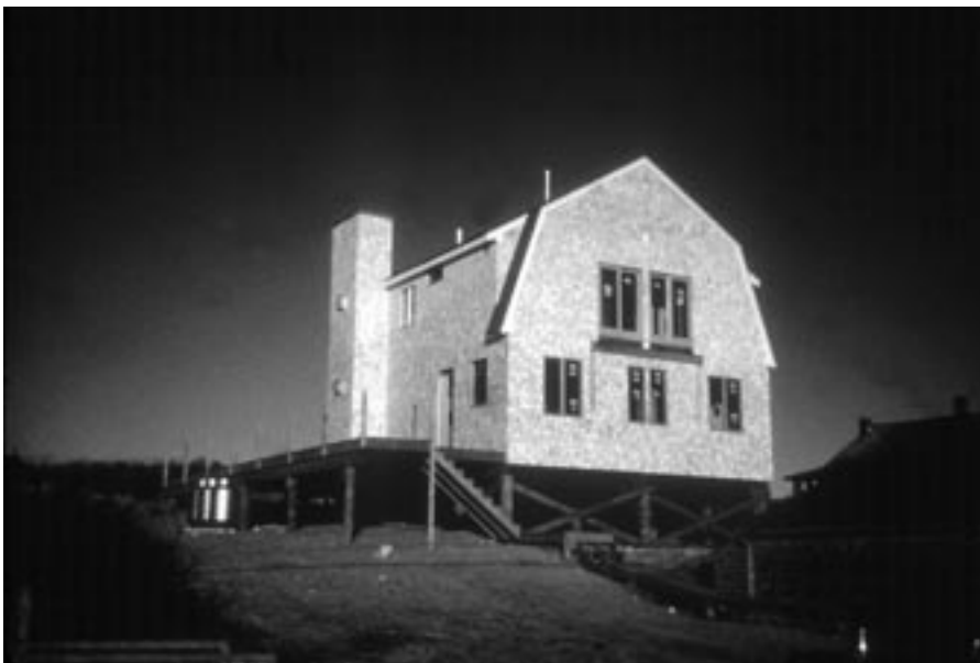
Figure 14. House elevated on open pile foundation
