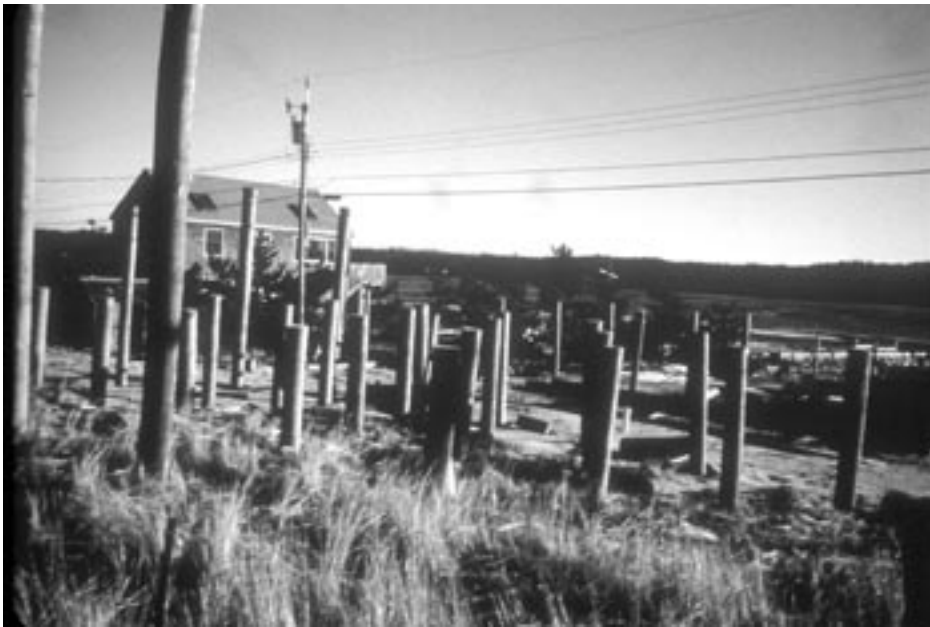
Figure 16. Coastal storm damage along Sandwich shore following the October '91 Nor'easter
