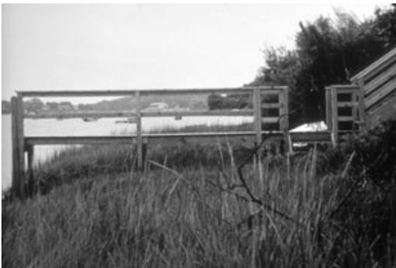
Figure 22. Elevated saltmarsh walkway
