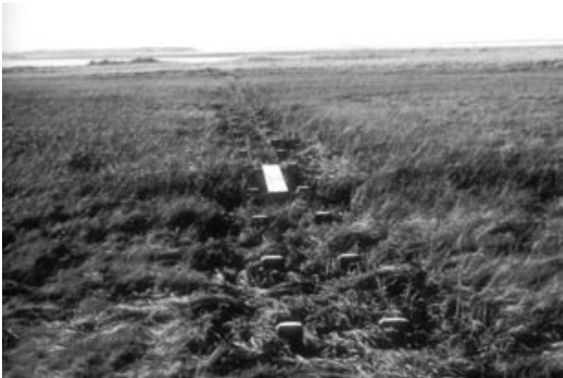
Figure 21. Stub pilings used for saltmarsh walkway
