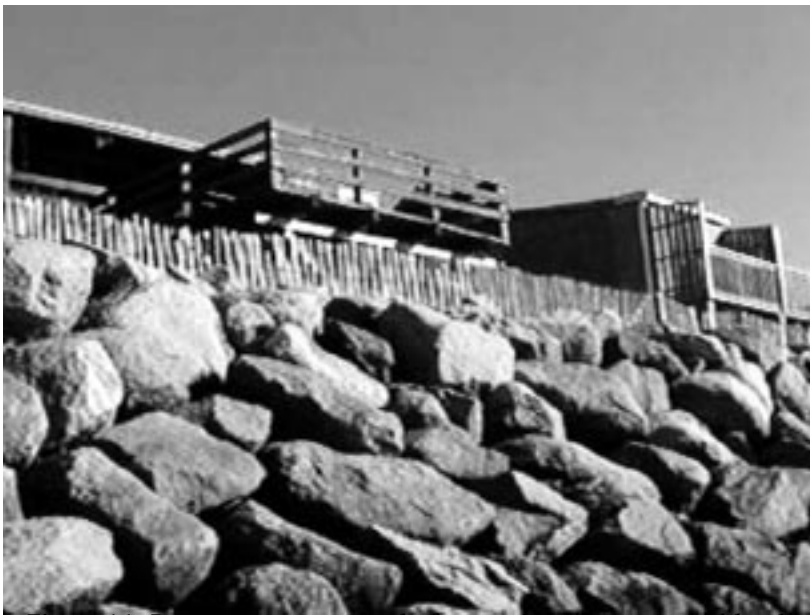
Figure 11. Revetment constructed of stone riprap on a coastal bank
