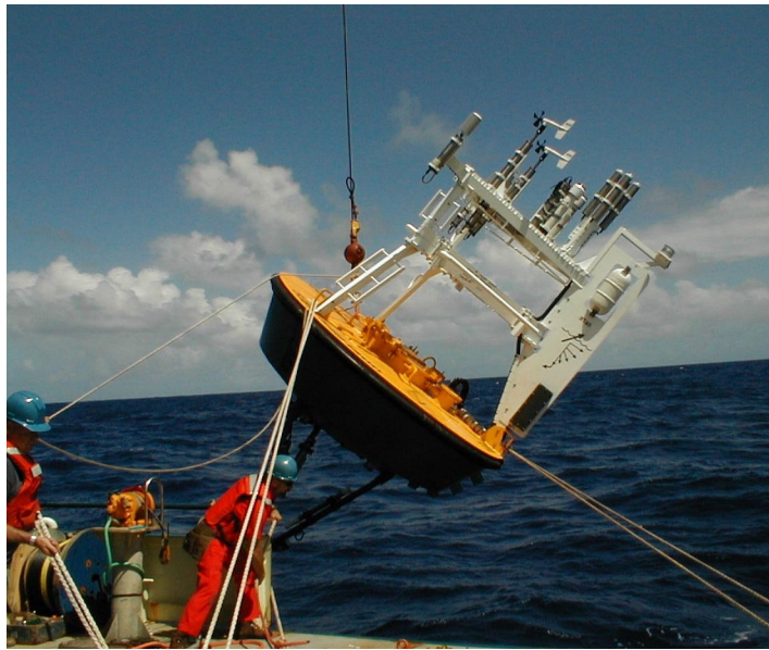
Figure 24: Positioning of quick release hook (attached to the crane's whip) and slip lines during the buoy deployment phase.
