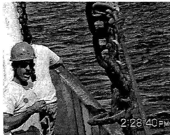
Picture 21. Attaching bottom of shot of four links of 2\frac{1}{4} " chain to 1" crown line chain.
