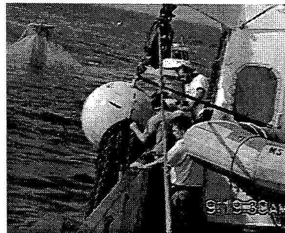
Picture 38. The Northwestern corner grid buoy with riser line attached. The line is being attached to the fish cage in the back left while the Galen J. stands by.
