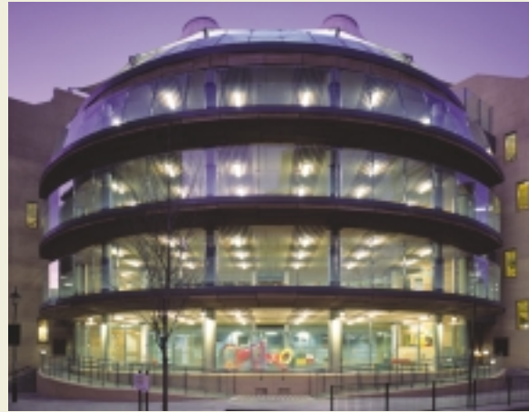
Credit: Building Design Partnership, Architect/Engineer. Photograph, Martine Hamilton Knight
