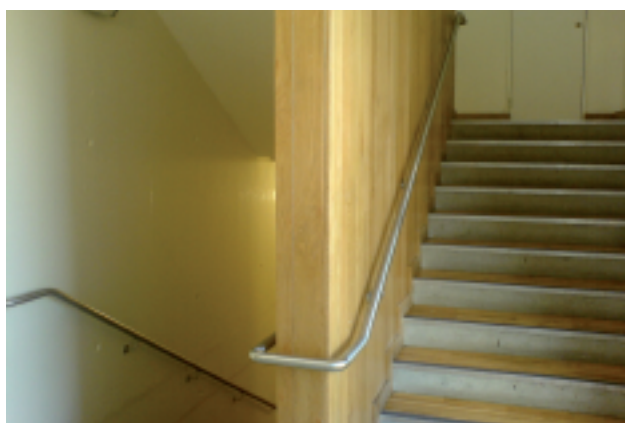
▲ Above timber clad wall between flights instead of a balustrade, with matching finish to treads
