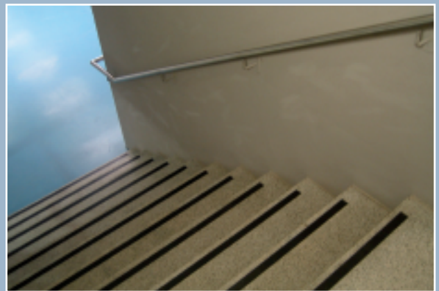
▲ Above carborundum strips set into pre-cast terrazzo treads on pre-cast concrete stair and an in-situ concrete central wall between flights instead of a balustrade
