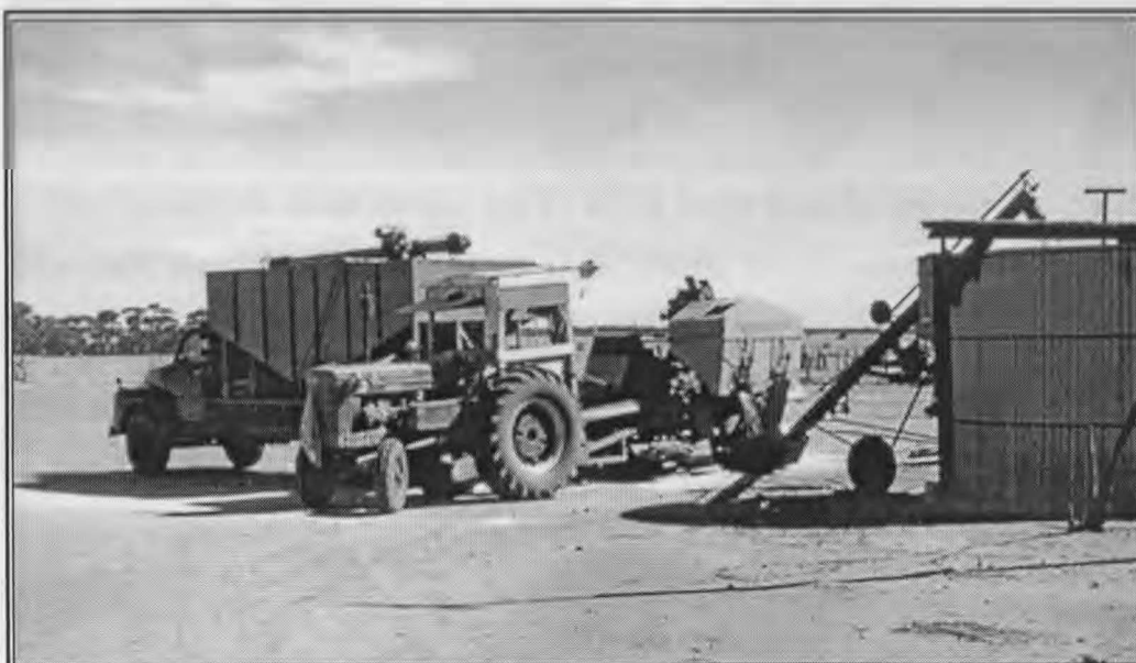
Dirty oats: grain runs from the truck bin down a corrugated iron chute and through the Horwood Bagshaw again. The cleaned grain pours from the yellow bin into a hopper and is augered into the round bin. November 1960.
