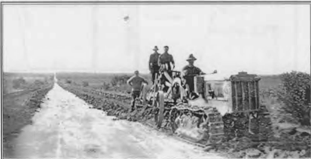
Hec Rhind on his Holt 2-ton crawler tractor, repairing a typical dirt road with an Adams grader near Koorda in the early 1930s. The bitumen began a hundred kilometres west of Wylie. Click the image for the Crawler Tractor page.
