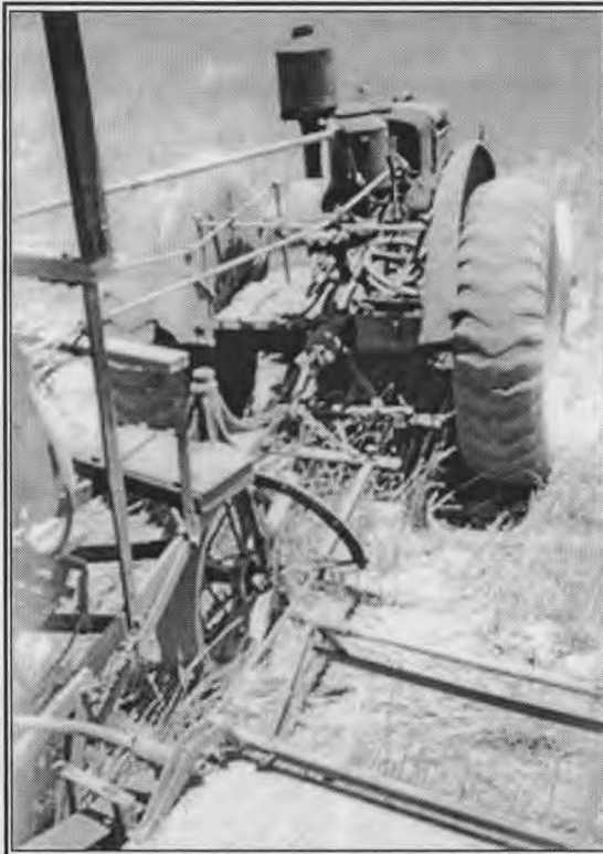
Remote controls on the Lanz HR tractor. December 1947.
