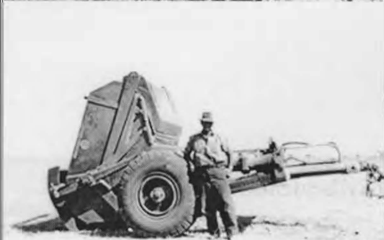
The dam contractor excavating the 3,000 cubic metre dam with an International TD18 bulldozer and hydraulic scoop in 1954.
