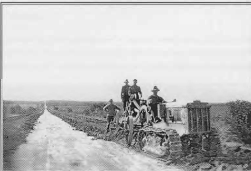
Hec worked for the Koorda Road Board during the Depression, pulling an Adams grader with his Holt. Note the crank handle. Early 1930s.
