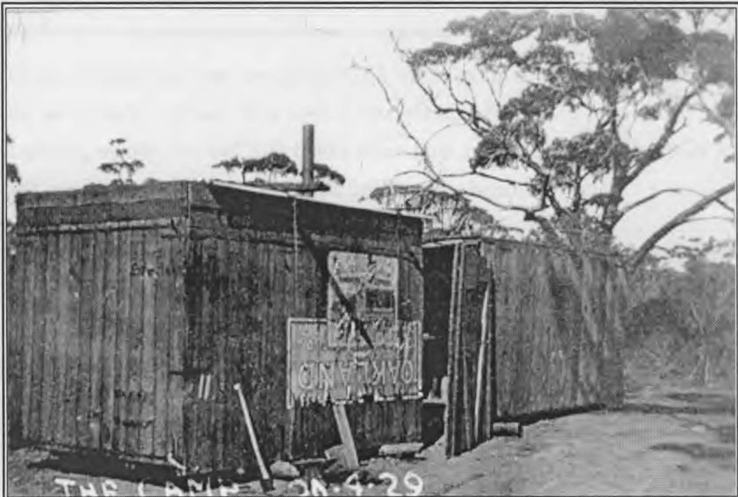
The closest crate is the kitchen, with a tin roof held down by poles wired down to logs under the crate. The chimney is connected to a wood stove. The far crate is the bedroom. Kulja, 20th April 1929.
