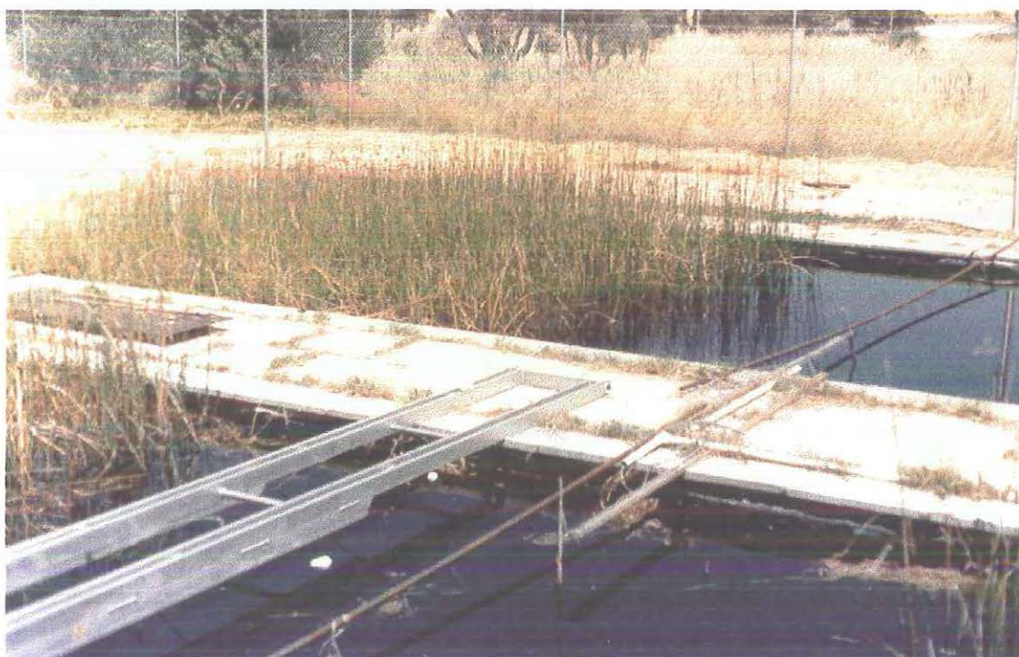
Plate 2.1 Hammond Road CWS (November 1999) showing portions of Cell 2 (front) and Cell 3 (back). Vegetation of Schoenoplectus validus can clearly be seen. Each cell is divided by a concrete walkway (centre) by which each experimental cell can be accessed.
