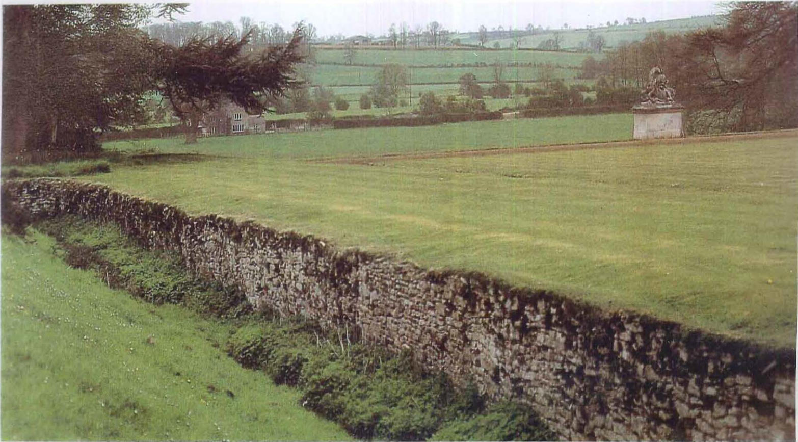
Figure 13: William Kent, The Ha-Ha , (Ogrin, 1993, p. 151), c. 1730, architectural landscape feature comprising a sunken ditch, stones and a fence at the bottom, Rousham, Oxfordshire, England.
